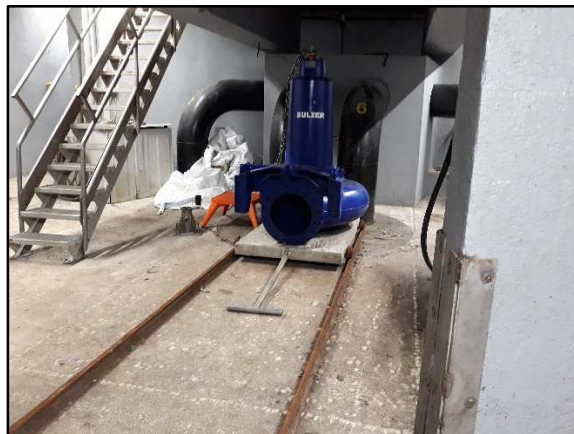
Paviment i carril guia
